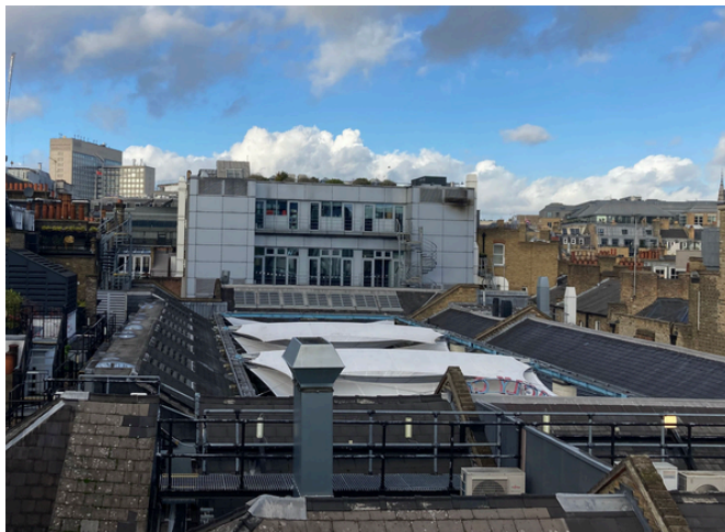
Existing temporary canopy above Kingly Court
